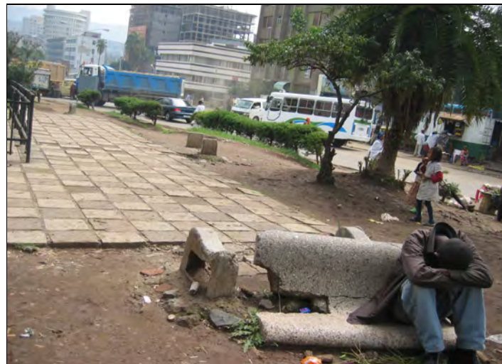
Fig.69. People using broken concrete seats at Leghar Park.
