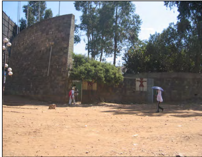
Fig.48. The Public toilet at Meskel Square which is part of Polony`s design of the square.
