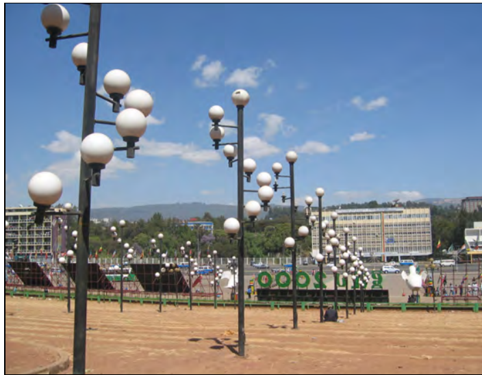
Fig.53.New lighting fittings at Meskel square
