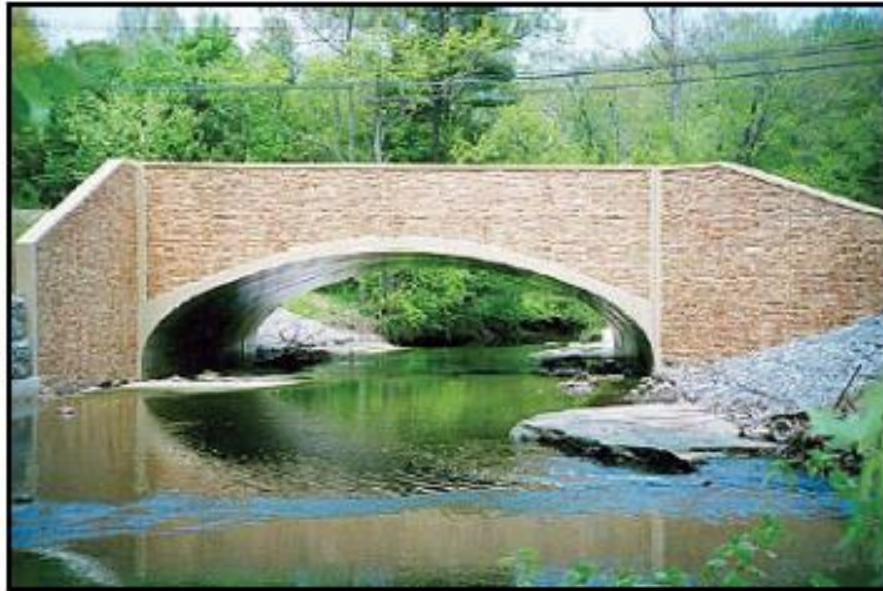
Figure 3.21: Typical example of an Open-Bottom Culvert with rounded top
