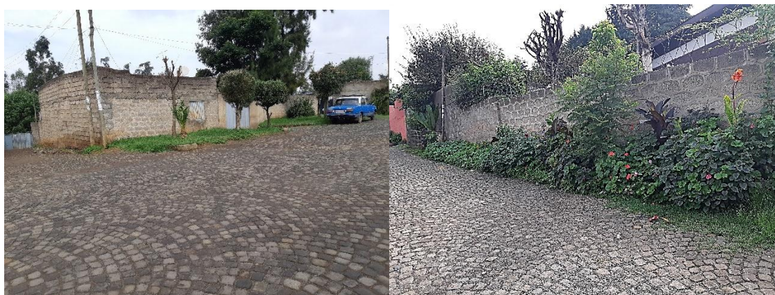
Figure 6 Cleaned cobblestone roads
