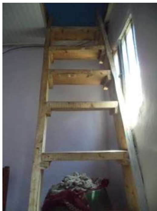
Figure 5-38 extension leading to blocking of openings
