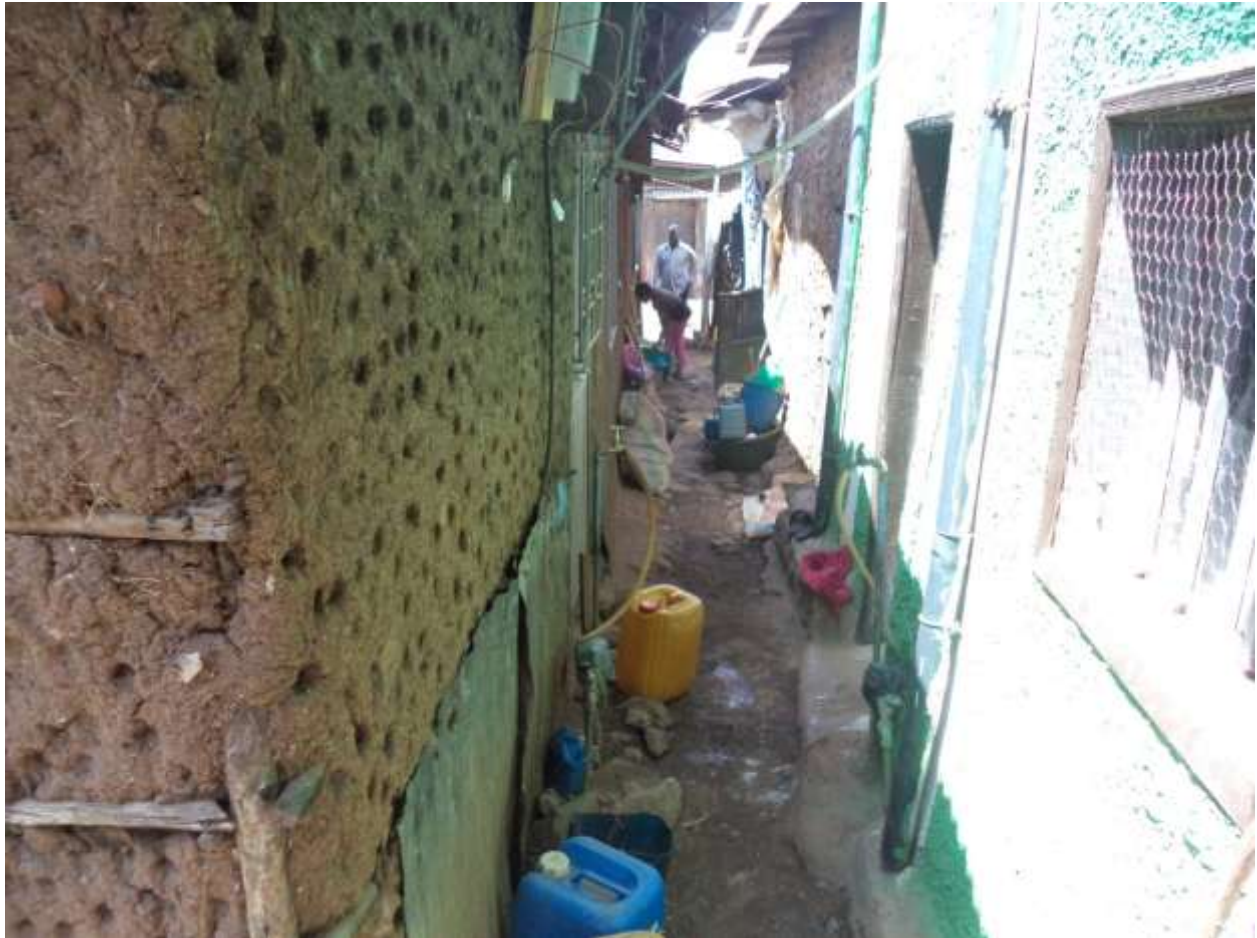
Figure 5-24 HBE operators house showing scarcity of open space
