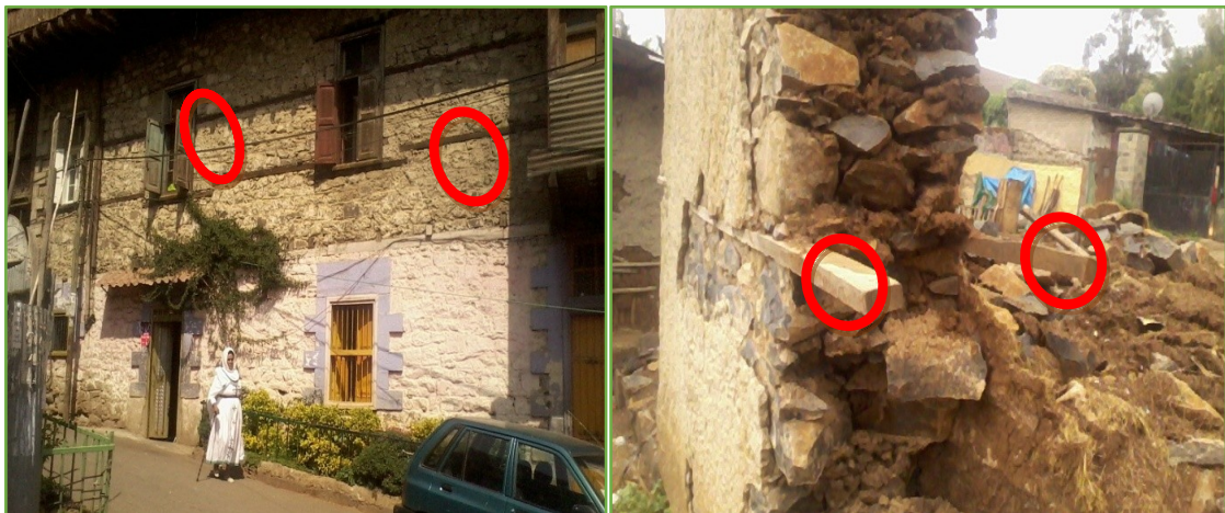
Figure 4: Timber laced building existing and demolished
