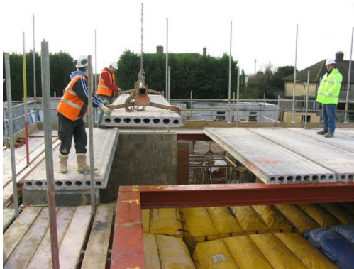
Figure 2.53. Installation of pre-tensioned slab (Spanwright, 2023) – Left and A suspended slab with post tensioning cables laid in position (Builderbill, 2012) – Right
