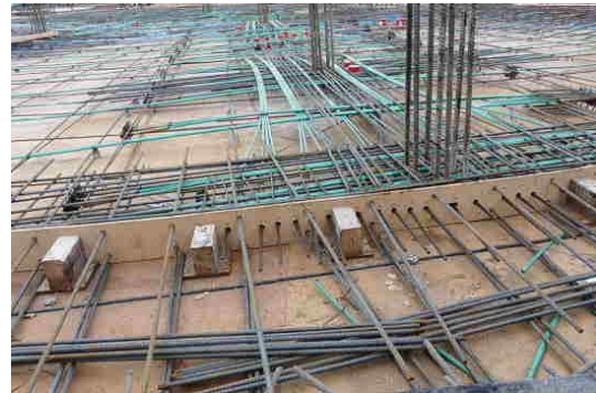
Figure 2.53. Installation of pre-tensioned slab (Spanwright, 2023) – Left and A suspended slab with post tensioning cables laid in position (Builderbill, 2012) – Right
