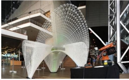
Figure 2.77. Daedalus Pavilion Measures 5m Wide X 5m Deep X 4.5m High, And It Consists of 48 Pieces That Are 3D Printed Using a KUKA Industrial Robot (Parametrichouse, 2023).
