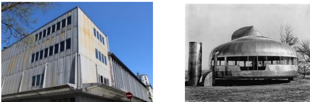
Figure 2.65. Facade to the offices of the “Maison du Peuple”, Clichy (F), 1939, Jean Prouvé – left and Prototype of a “Dymaxion Deployment Unit”, 1929/45, Buckminster Fuller - right (Herzog, 2004)
