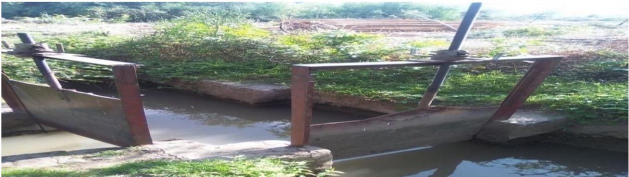
Figure 3. 3: Functional division box with gates
