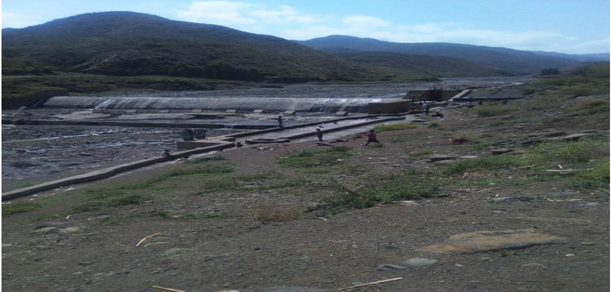
Appendix figure 7. 10: The diversion structure (weir)
