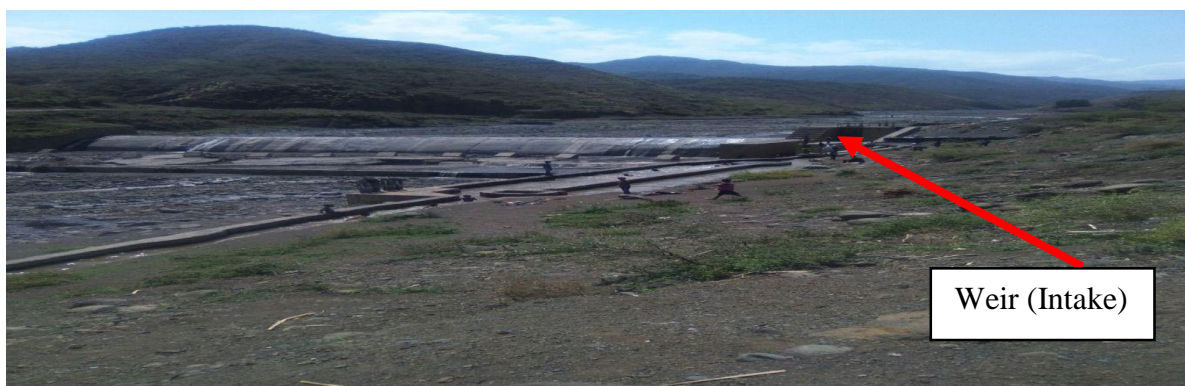
Figure 3. 2: Golina irrigation headwork structure
