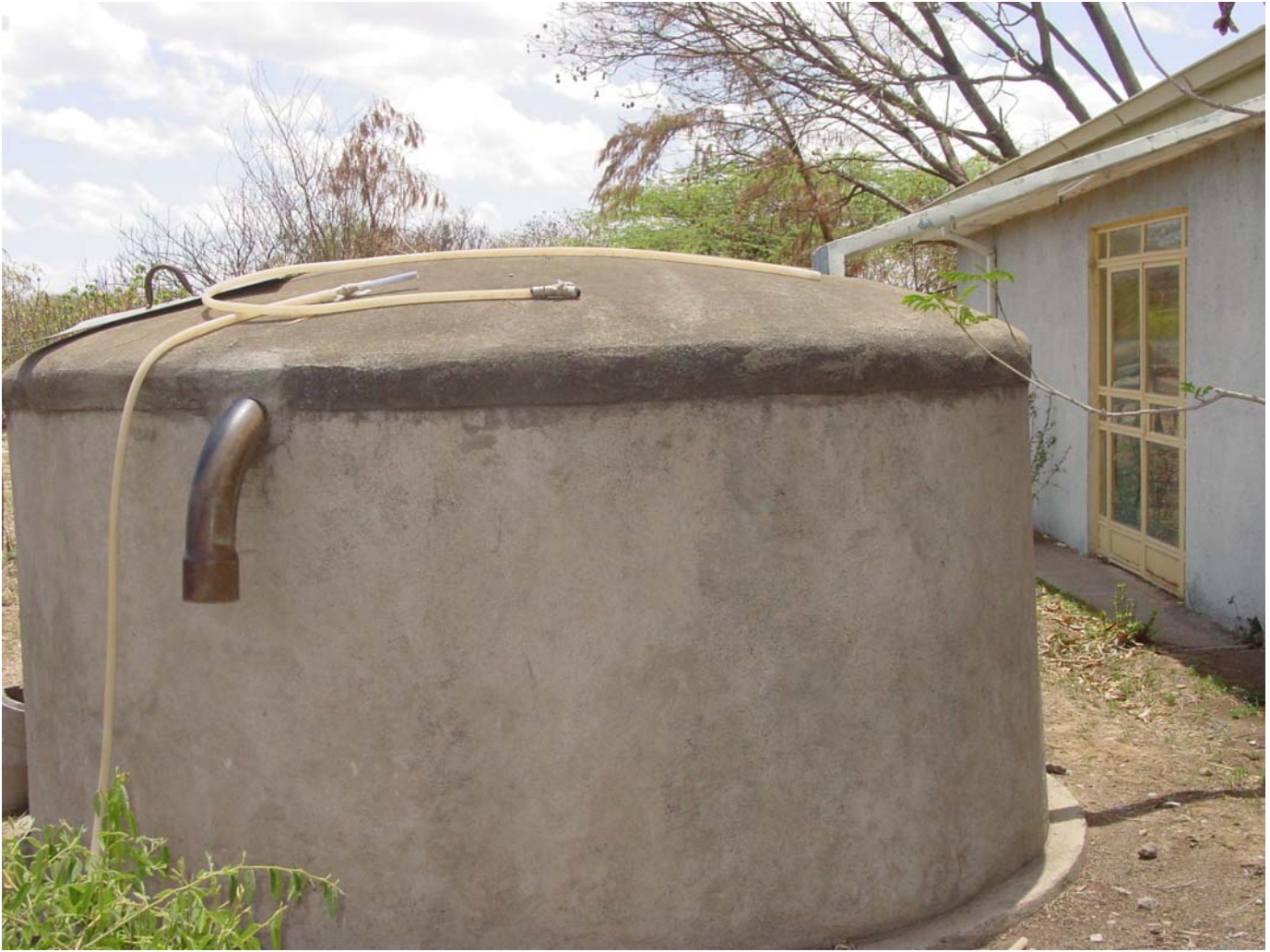
Picture 5b: Roof Top Water Storage in Alage
