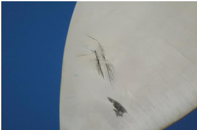
Leading-edge erosion Adama wind farm I
