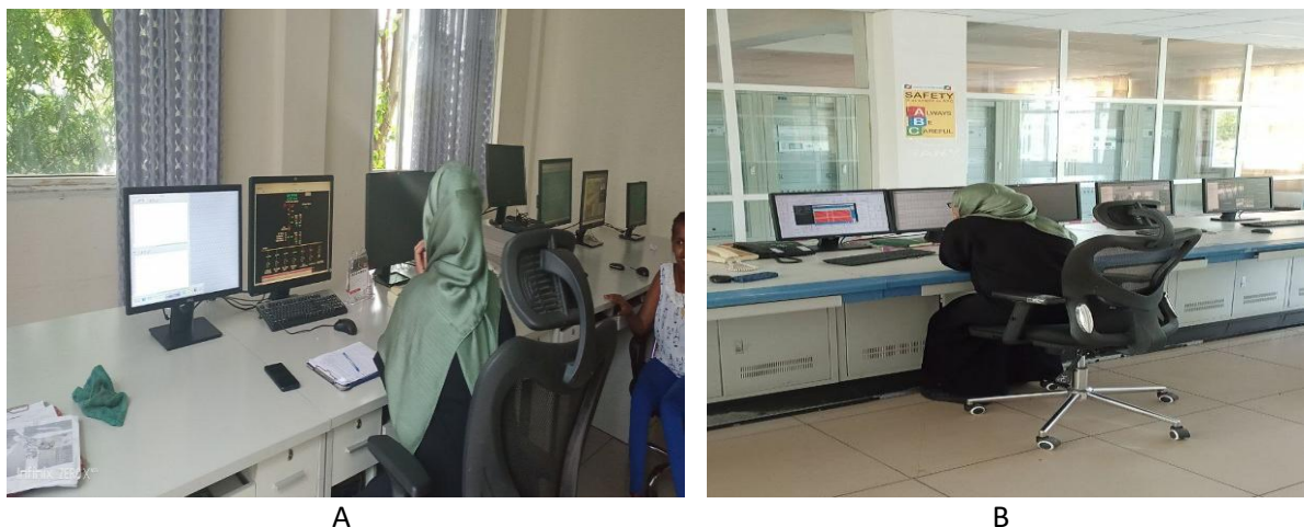
Figure 14 Adama I (a) and Adama II control room (b)
