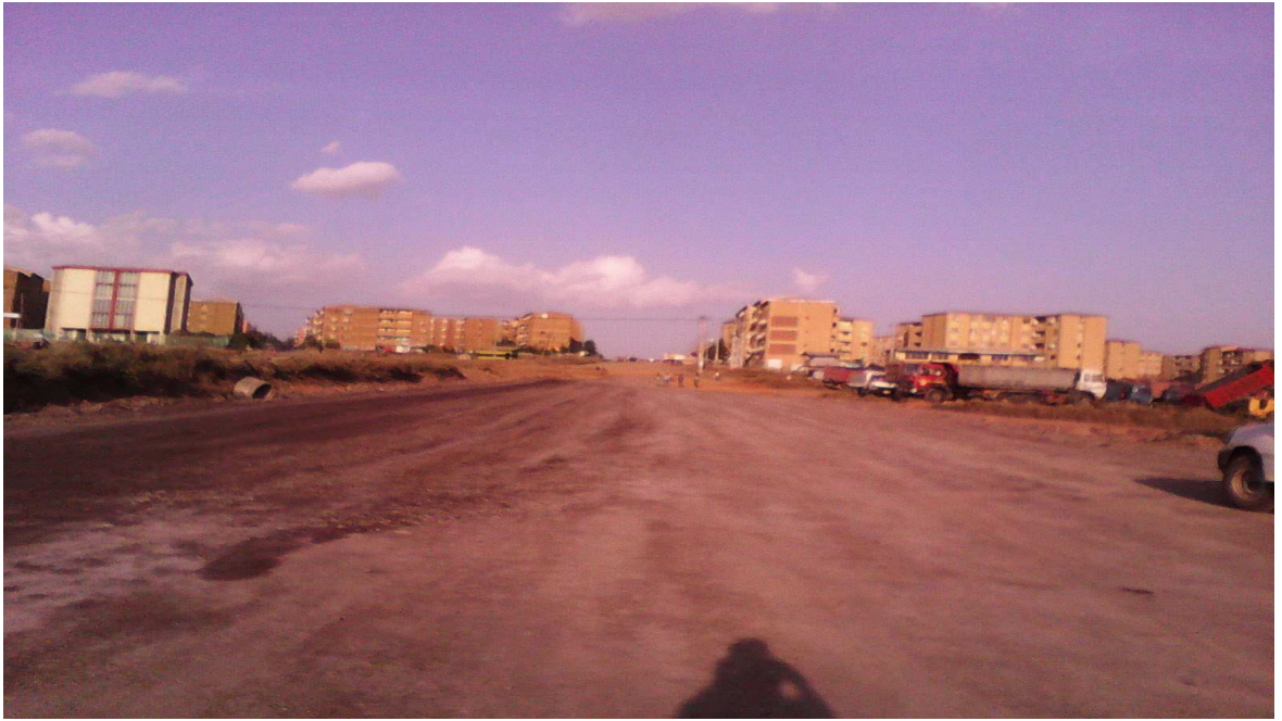
Fig.D-3 Finished sub-base layer of the road.
