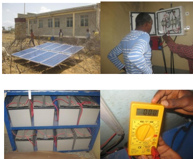
Figure 3.6: Adifetaw Health post in Tigray region . Inverter output is zero
