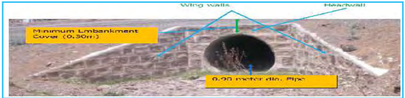
Figure 6.5: Proposed Pipe Culvert at Station 23+100
