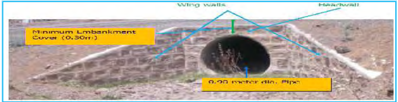
Figure 6.4: Proposed Pipe Culvert at Station 22+500
