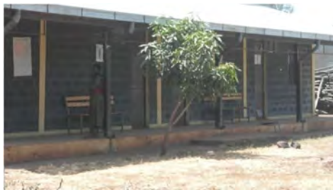
Fig5.5 Currently installed Solar panel for deck health center
