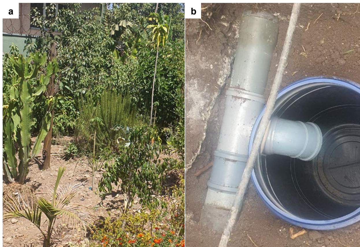
Figure 6.4: Sample picture of a) RG development on the field and b) RB installation
