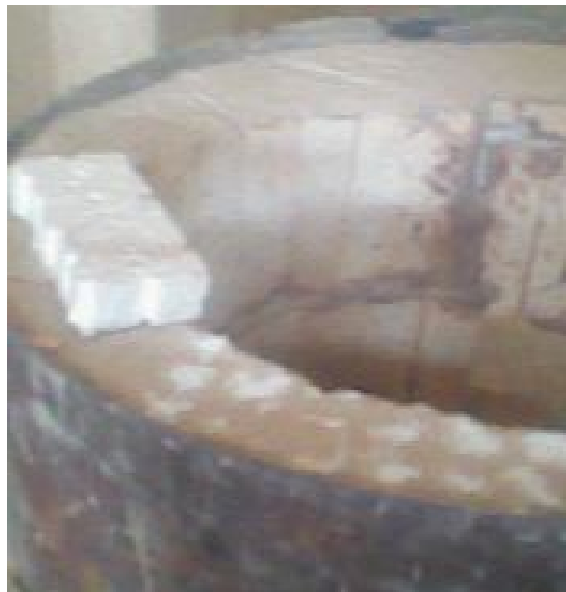
Figure4.6: Coal Firing Chamber Manufactured in TCF for Spray Drier
