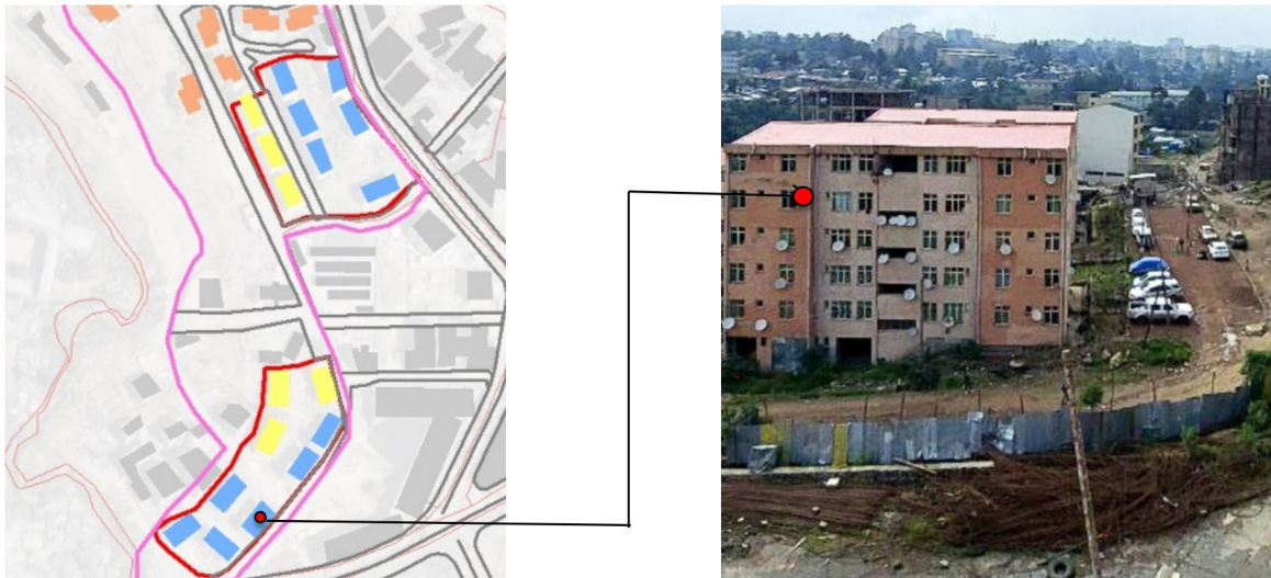
Figure 4.20: W/ro Sumeya Ali's one-bedroom housing unit location at lower Basha Wolde condominium
