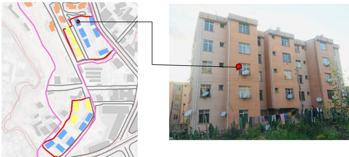
Figure 4.22: Sajin Werke Melaku’s one-bedroom housing unit at upper Basha Wolde condominium
