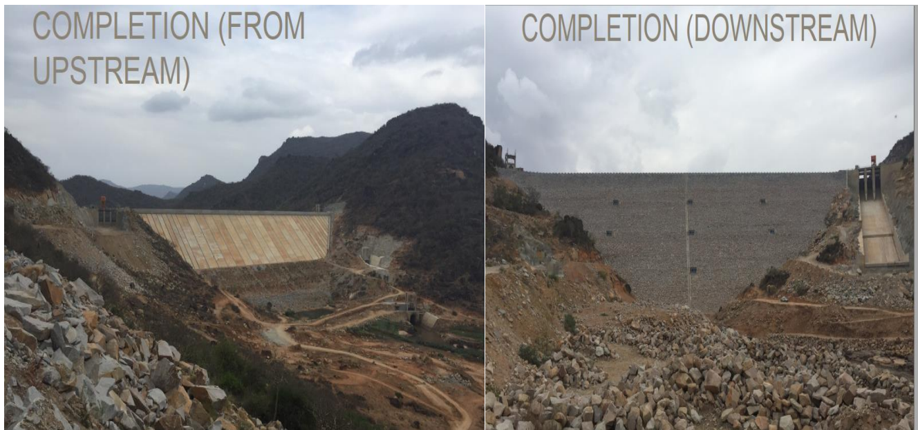
Figure 3-4 Upstream and Down Stream View [EEP March 2017]
