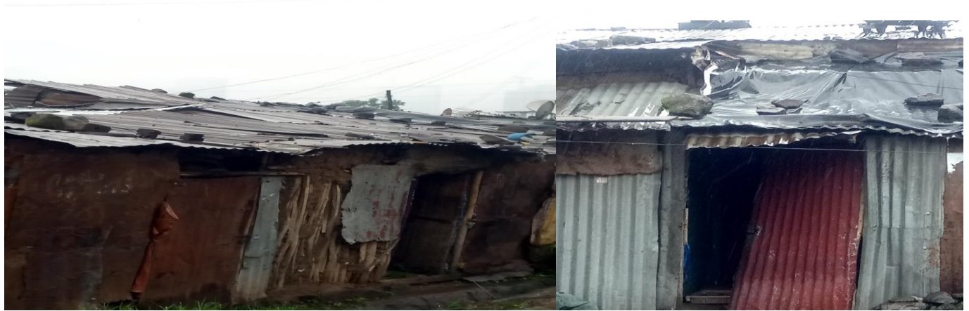
Figure 4.3 Housing conditions of UPSNP beneficiaries
