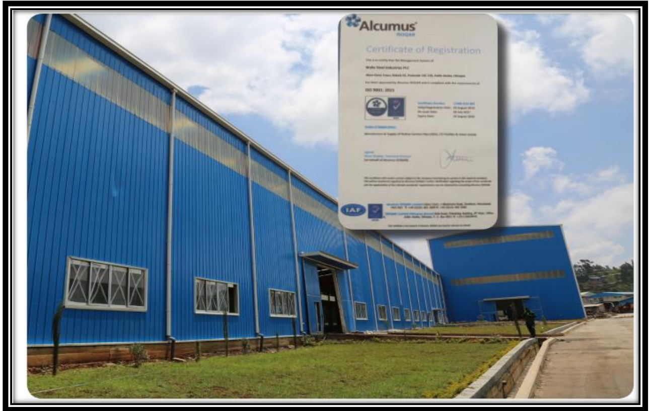
Figure 3-1 Part of Walia Steel Factory
