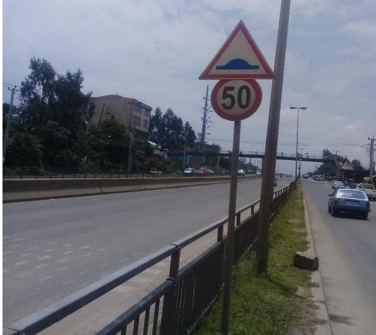
Figure 4- 11 Speed Hump Warning Sign
