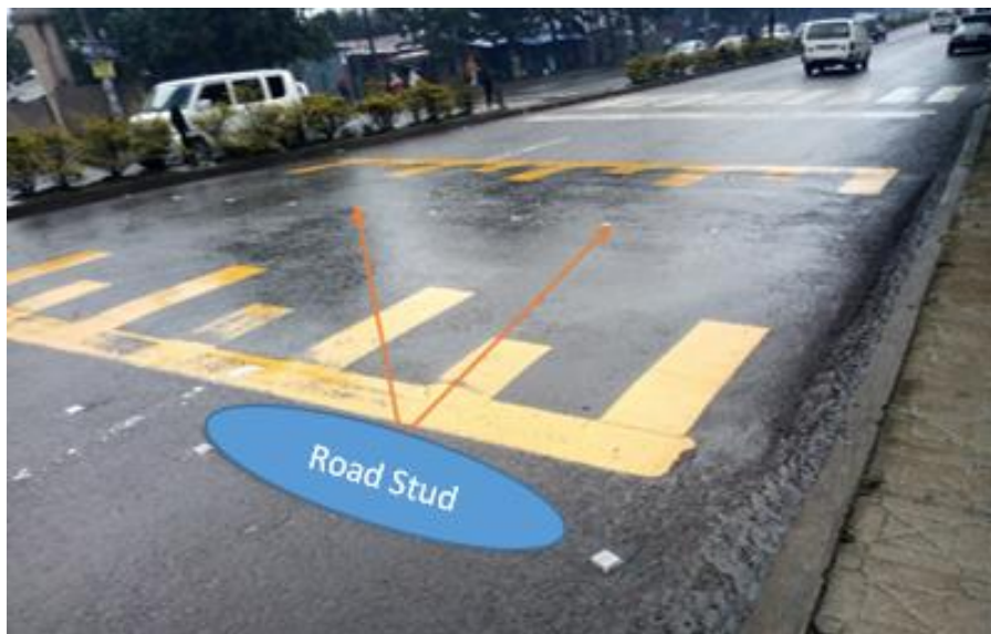
Figure 4- 18 Photo shows reflectors on hump
