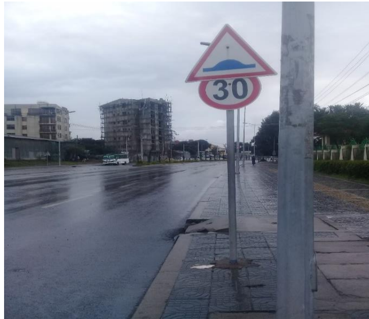
Figure 4- 20 Speed Hump Warning Sign
