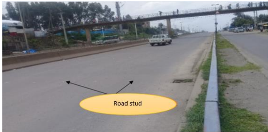
Figure 4- 14 Photo shows reflectors on hump
