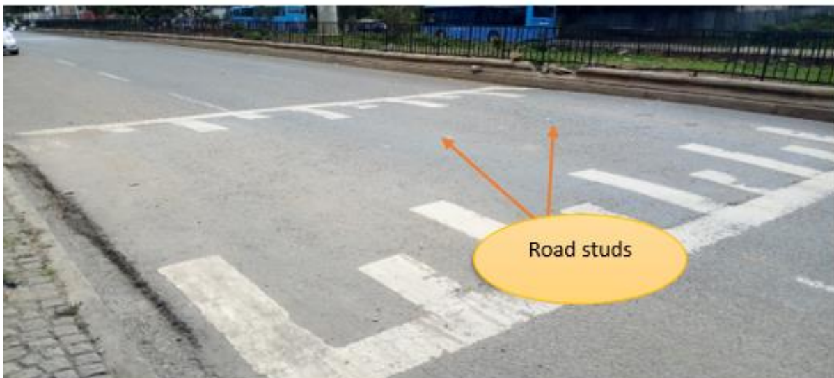
Figure 4- 9 Photo shows reflectors on hump
