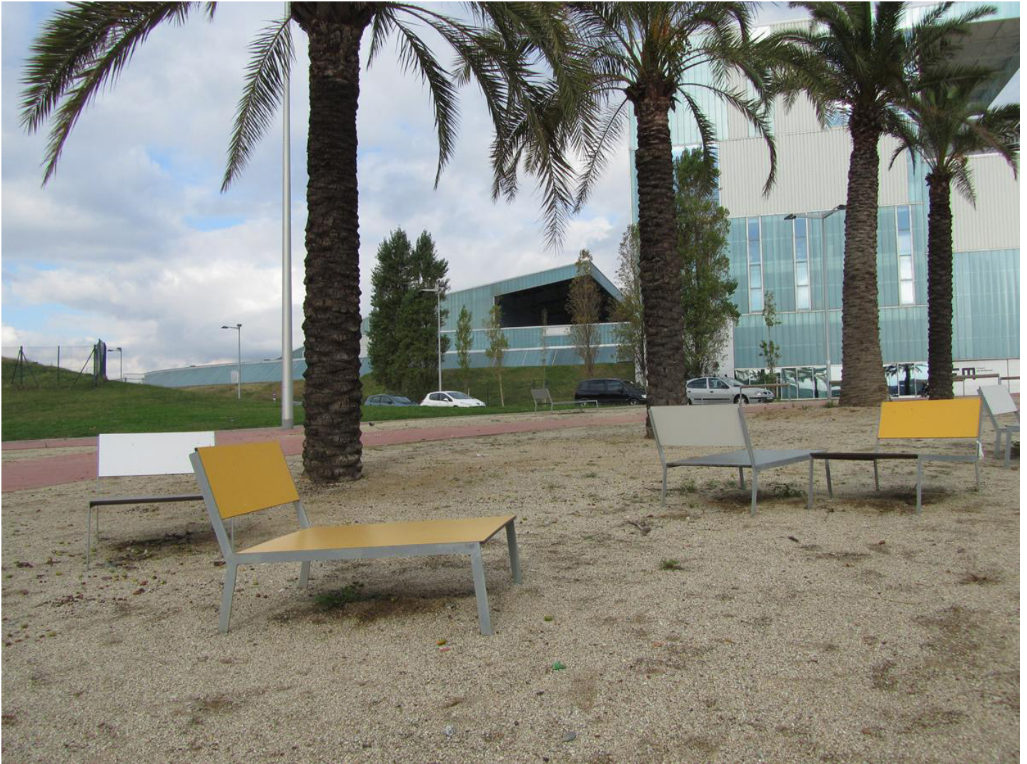
Figure 30 : ECO PARK waste to energy plant
