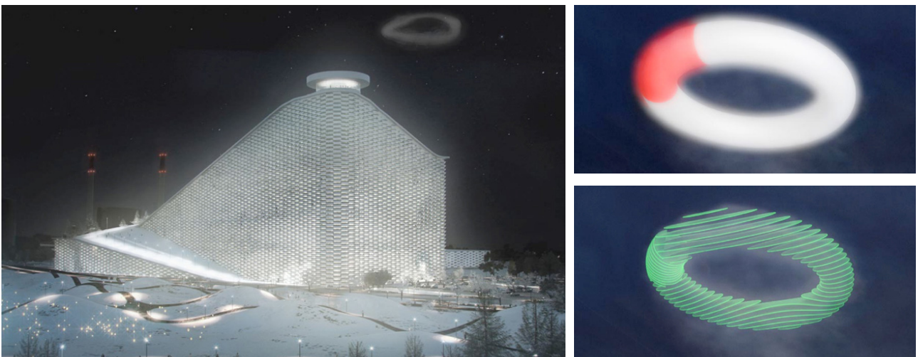
Figure 25 : Amager Bakke waste to energy plant projected laser light on smoke ring illustrating, in pie chart form, the quota of fossil CO 2 Source : www.Archdaily.com
