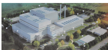
Figure 15: reppi WTE plant
