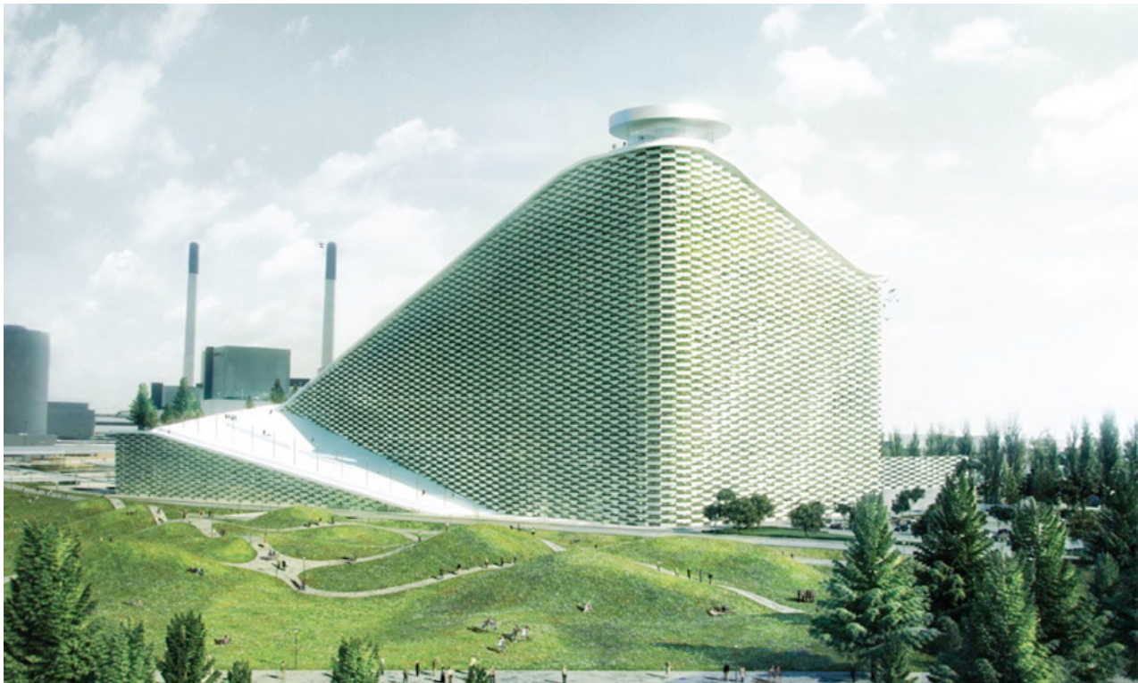
Figure 23: Amager Bakke waste to energy plant
