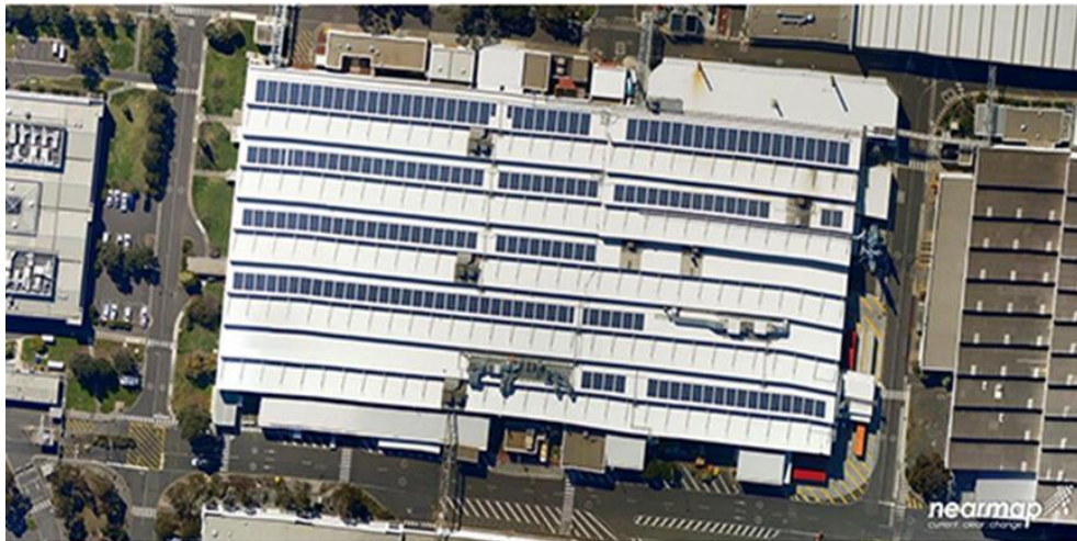
Figure 2.3 Illustration of Toyota 500kW Industrial Solar Power System [28]
