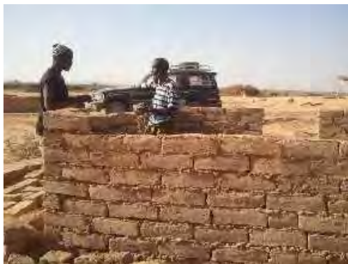
Photo.2.4 Manual compressed earth block from Silt - Sand Soil to construct houses.
