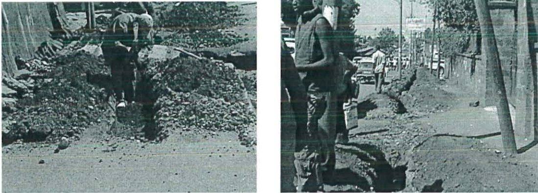
Figure 4.4 picture showing excavation of roads using “Doma” in the inner city
