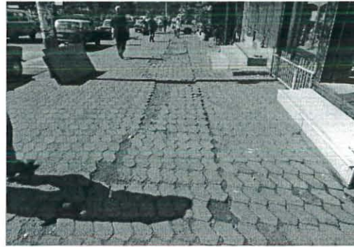
Figure 4.5, Picture showing road maintenance below the standard.
