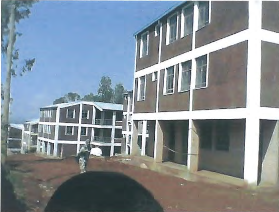
Figure.3.10: Photo showing Front side of Hostel site condominium Housing block
