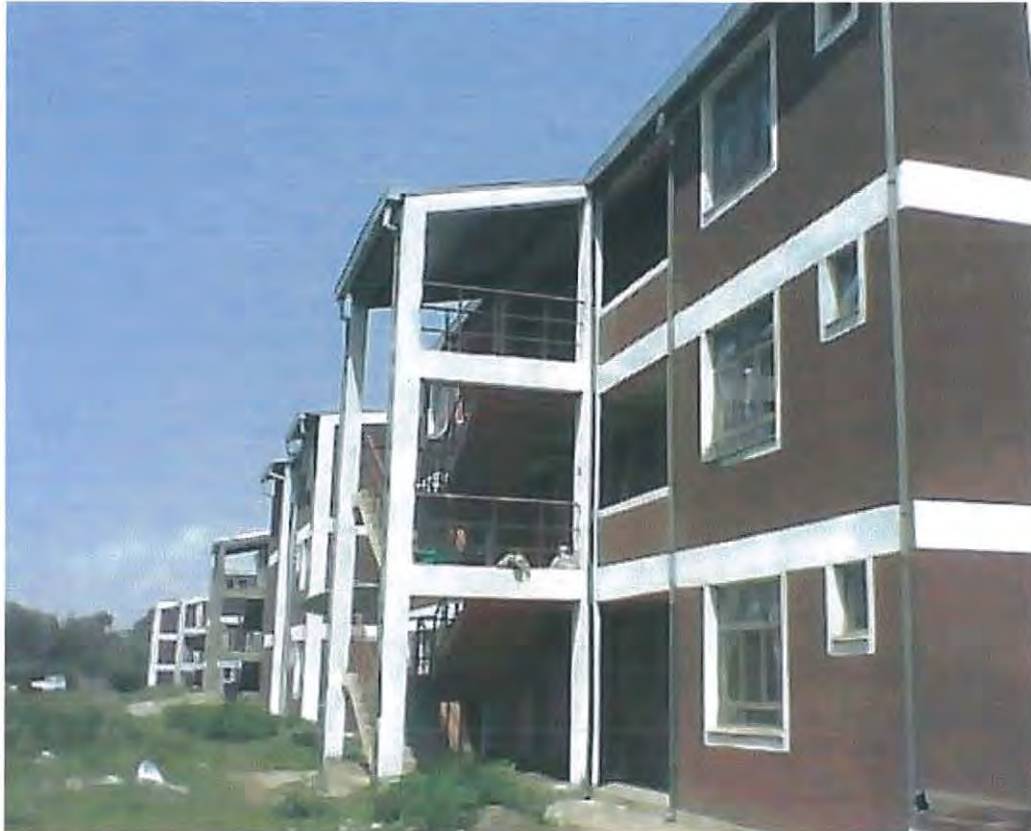
Figure.3.11: Photo showing one side of EDDC condominium site
