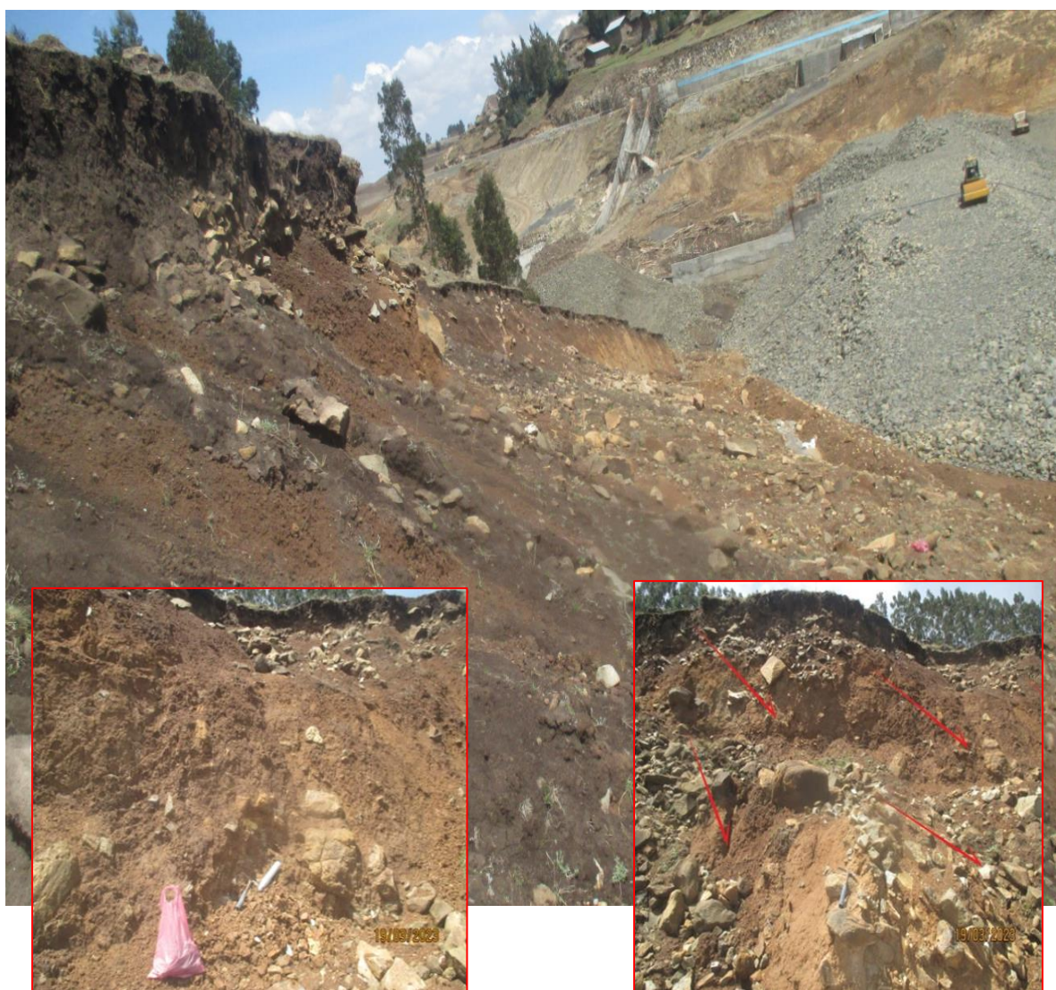
Plate 4-4: Field photo on critical slope section one (RS-3) on the left side of dam axis.
