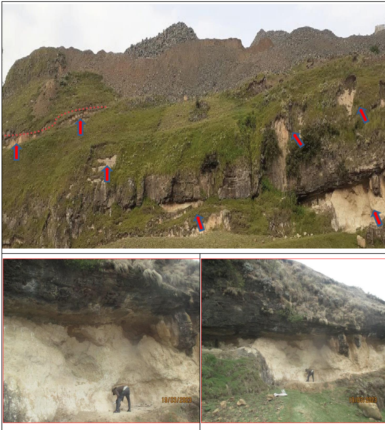
Plate 4-3: Field photo on critical slope section one (RS-2) below the quarry site one
