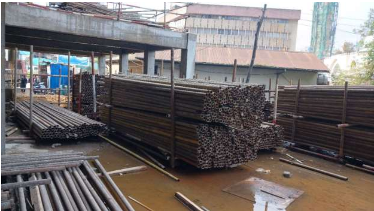
Figure 4. 9 Placing of H-frame and RHS (Taken by researcher)
