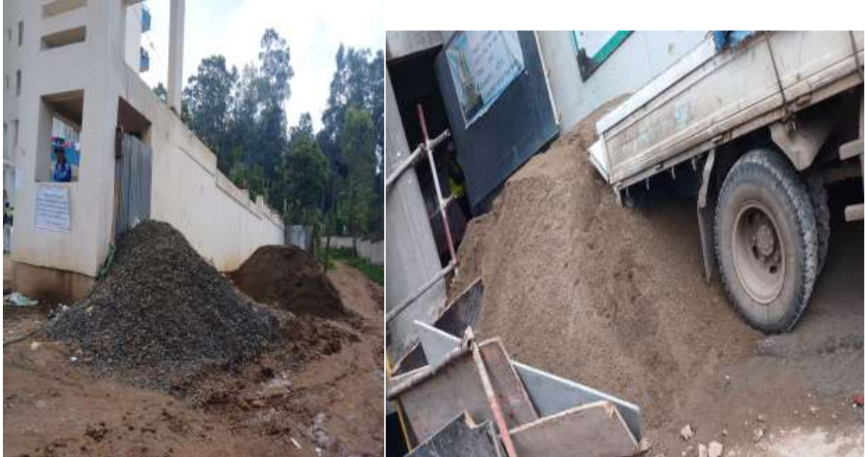
Figure 4. 10 Placing of aggregate and sand at site
