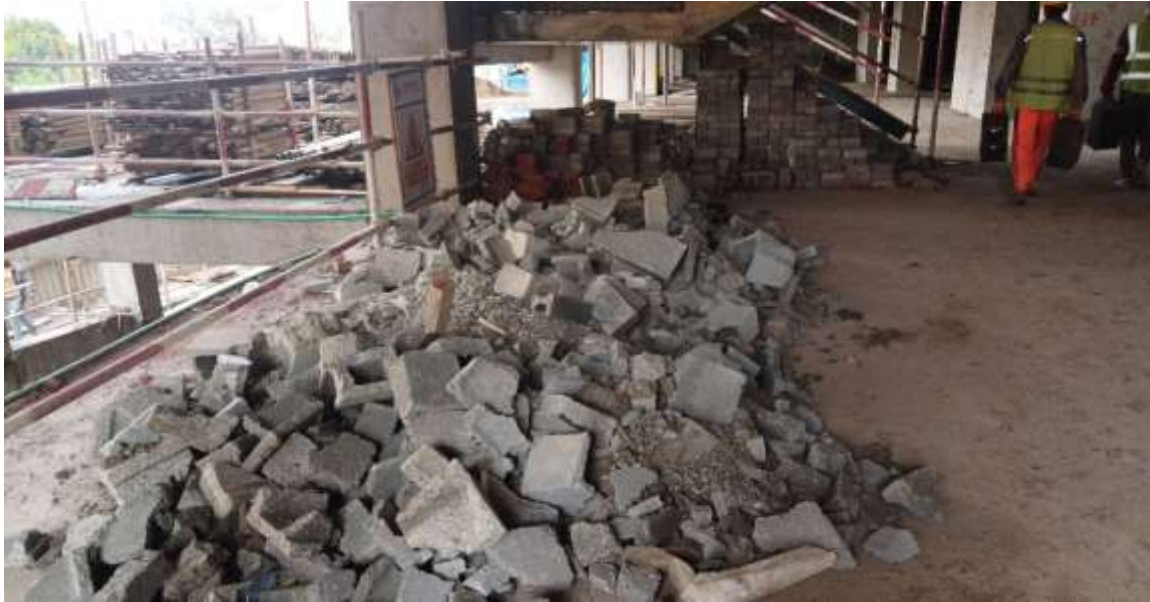
Figure 4. 12 Wastage of HCB material
