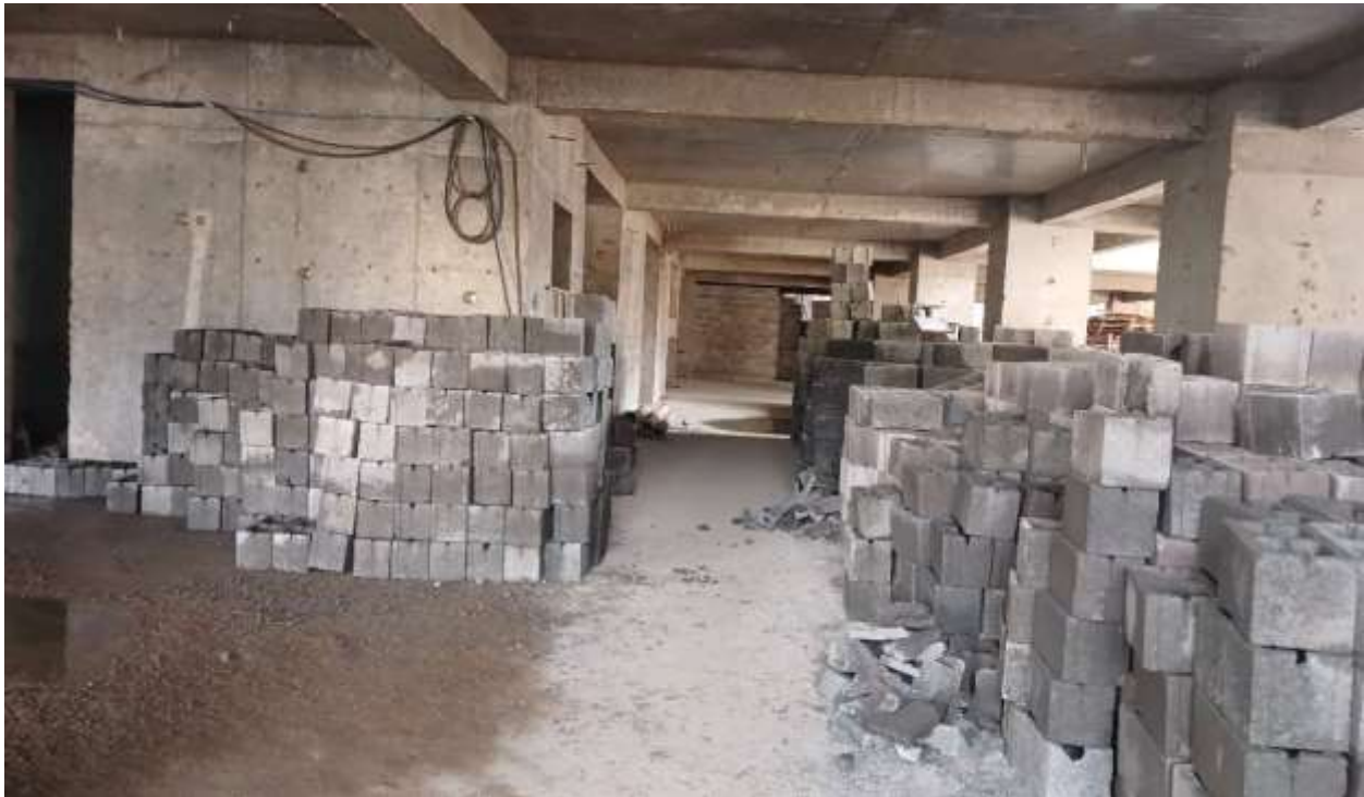
Figure 4. 11 Storage of HCB on site
