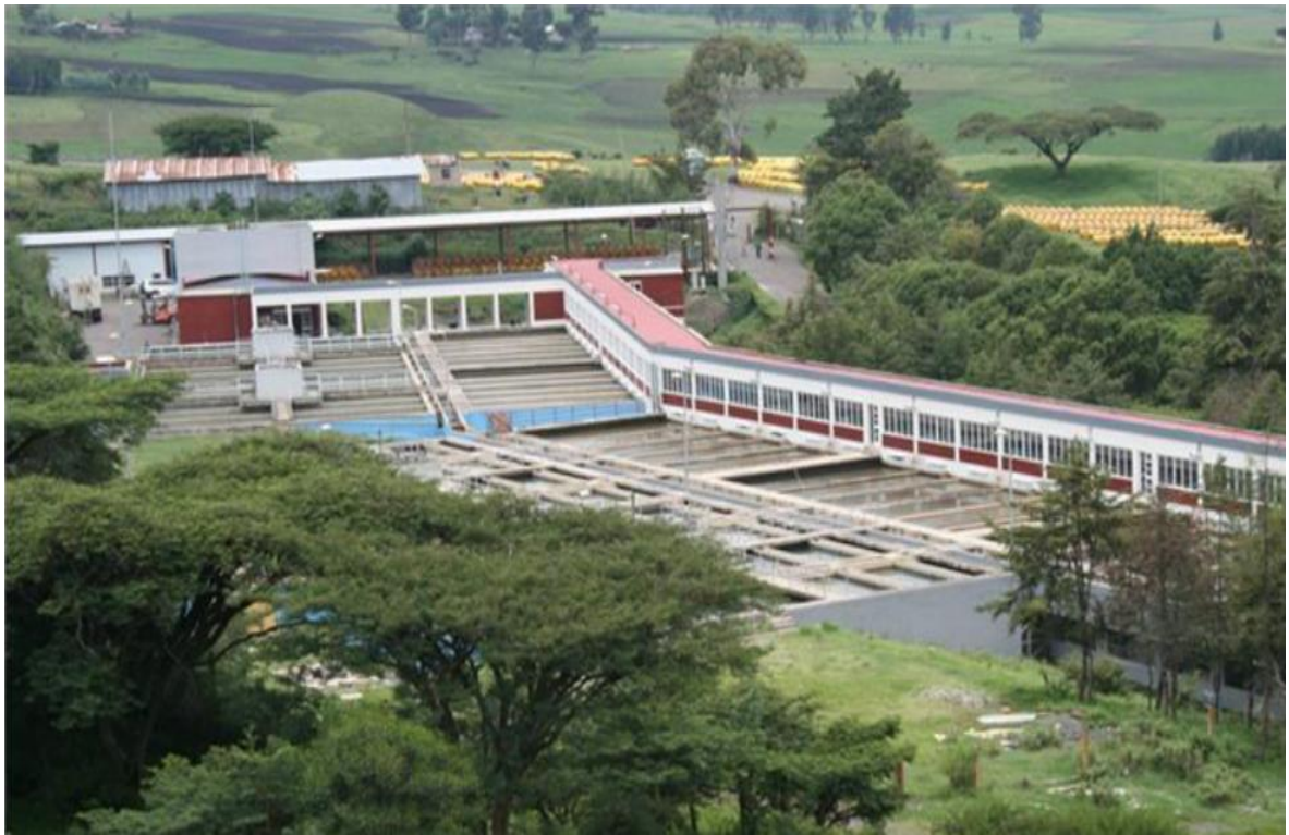
Figure 3: Legedadi Water Treatment Plant
