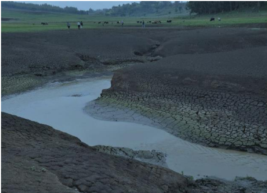
Figure 2: Siltation in the Legedadi Reservoir (2012)
