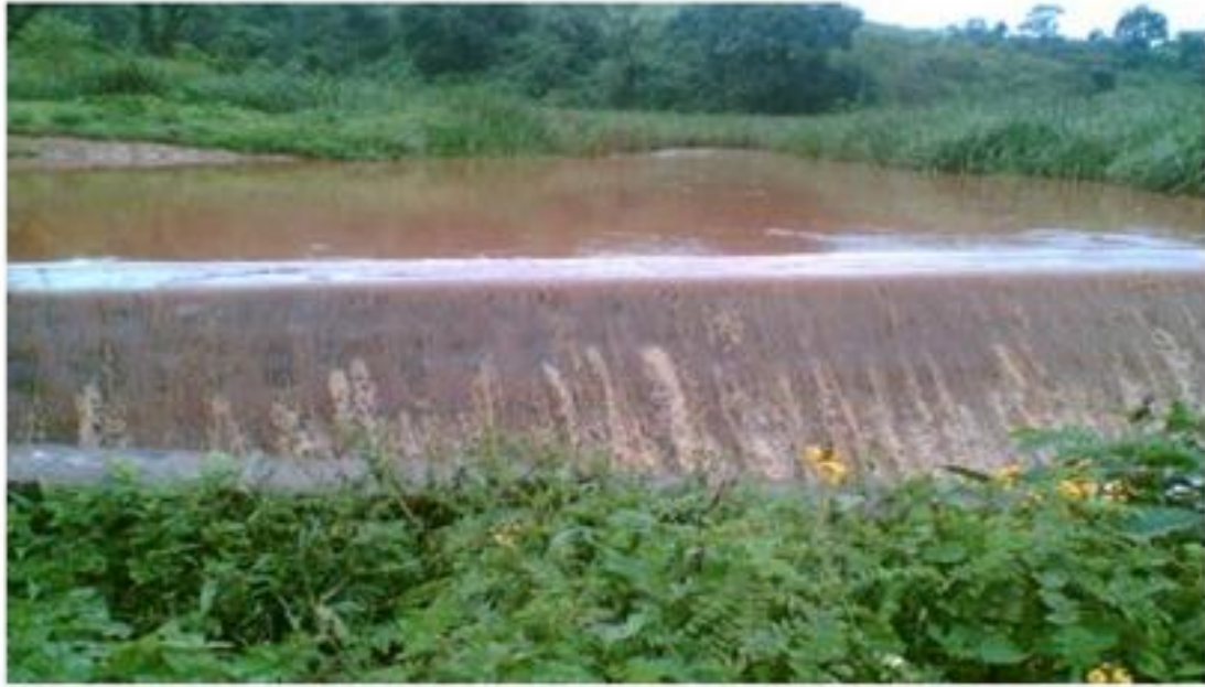
Figure 3-3: The intake weir structure of water supply source
