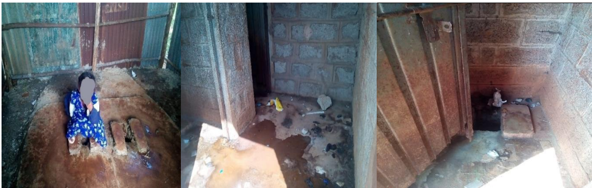
Figure 5. Appearance of Non-Standardized Preschool Toilets.
