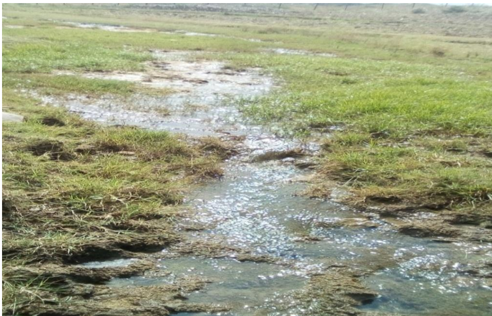
Figure 3. This picture showed that water loss through seepage from the main canal, in Semha village, March 2019 by Teklit Hagos (Photographer).
