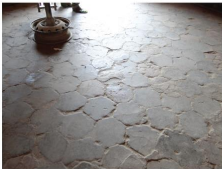
Cement Concrete hexagonal floor finish
