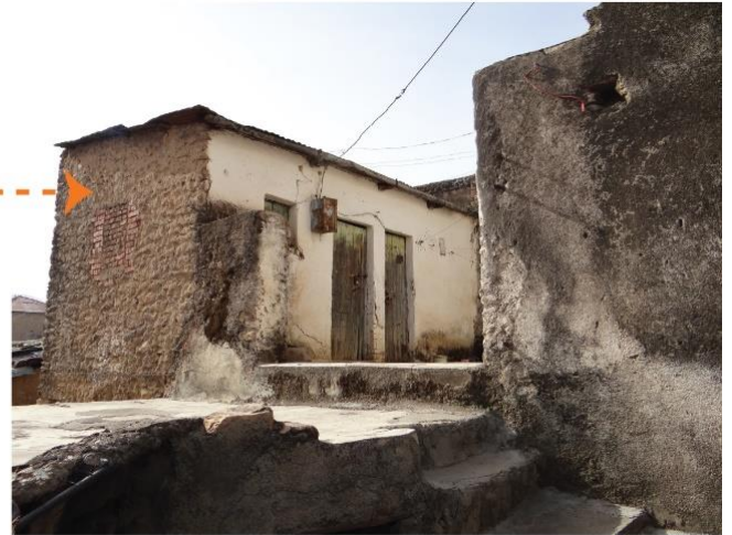
First Story Level rooms with Veranda.
