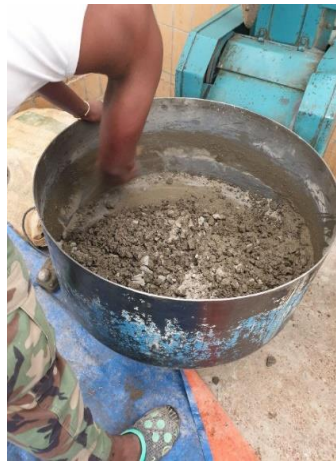
Figure 3-2: Mixing of concrete.
