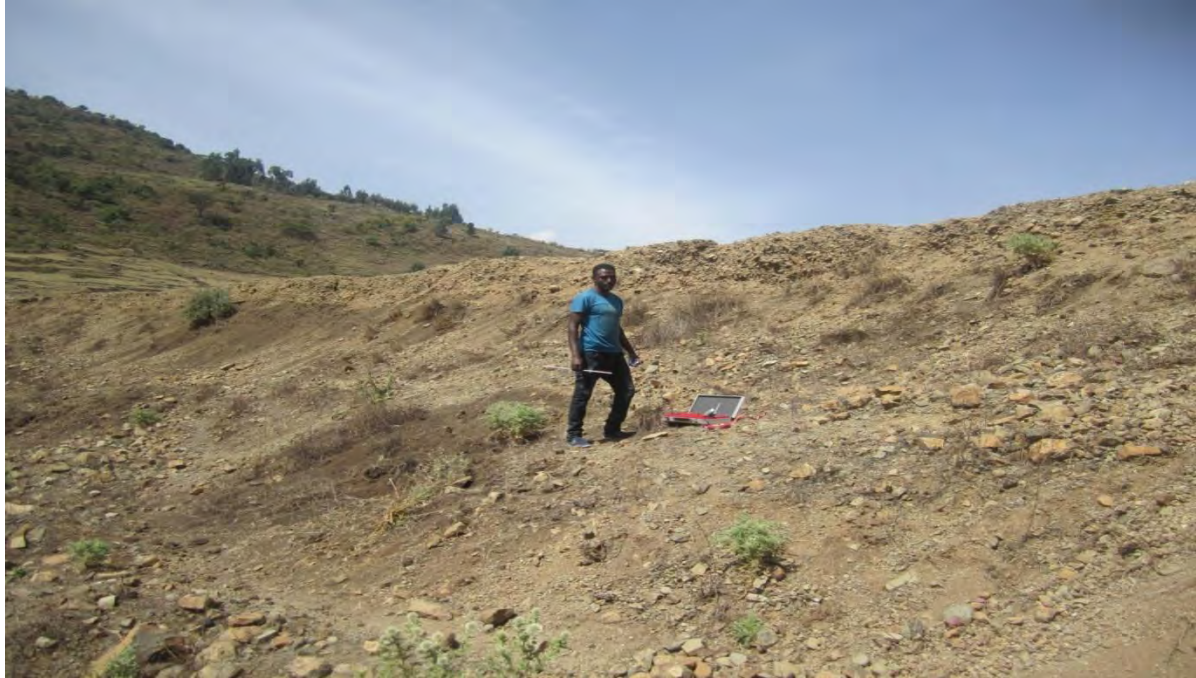
Photo-3 Slope face failure at the downstream
