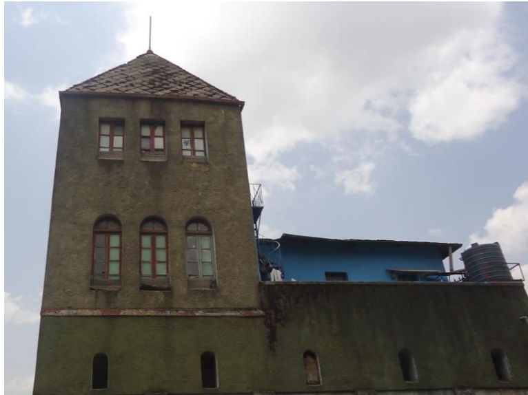
Figure 15: Arched transom and rectangular windows showing on the NW façade
