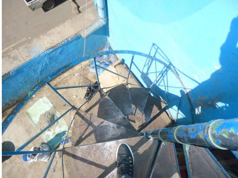
Figure 17: Metallic circular staircase located at the first-floor terrace
