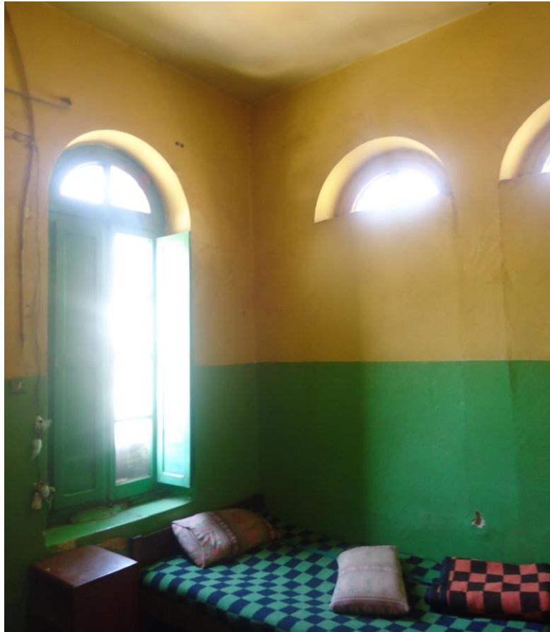
Figure 19: Wooden frame arched transom windows located in the first-floor bedroom
