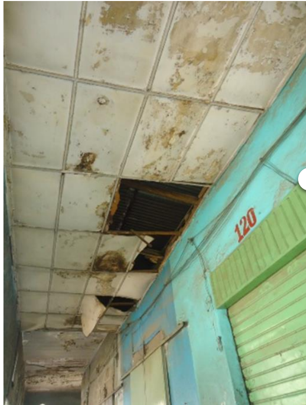
Figure 22: Ceiling damage located at the NW side of the corridor
