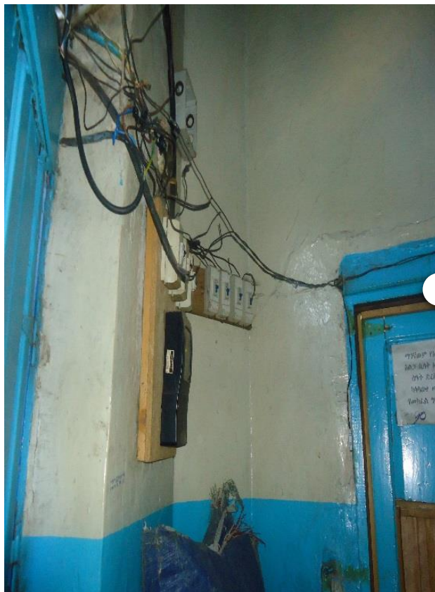
Figure 23: Poor electrical installation & exposed distribution board located at the left side of the entrance toward the first floor
