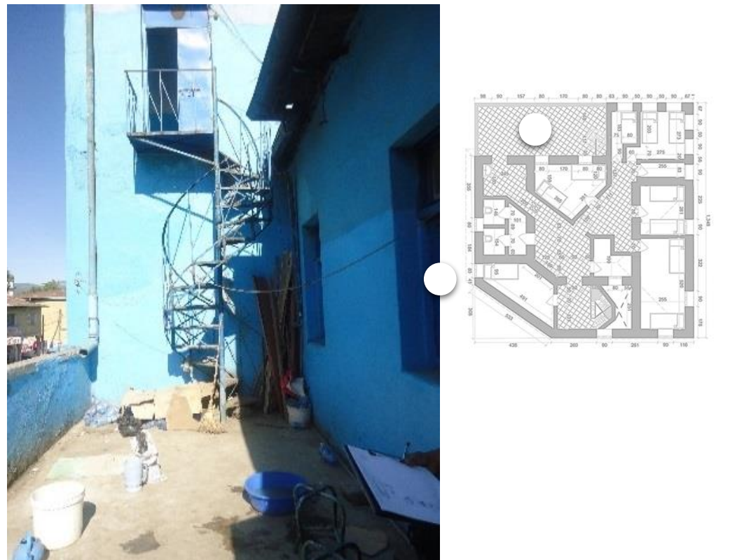
Figure 30: Picture shows the condition of the first-floor terrace
