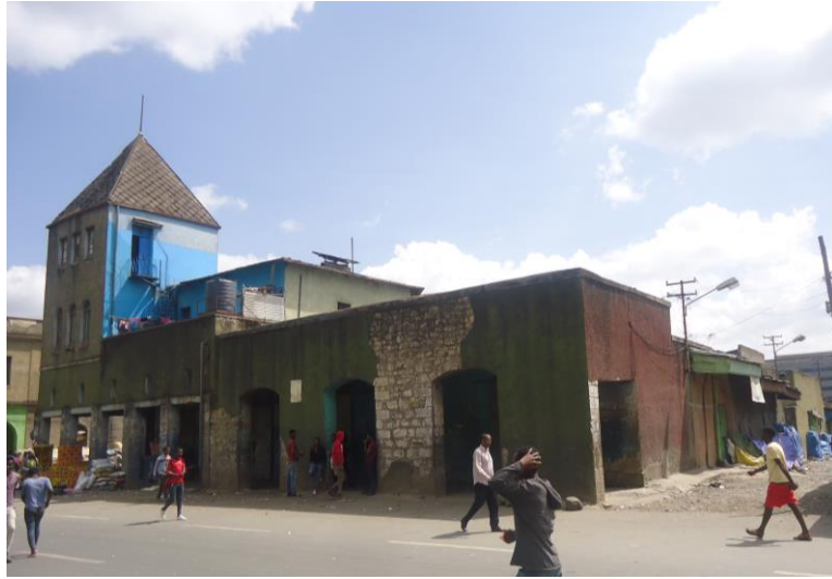
Figure 40: SW view showing the extended structure
