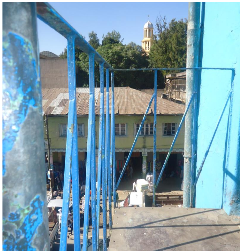
Figure 20: Metallic handrail located at the second-floor entry
