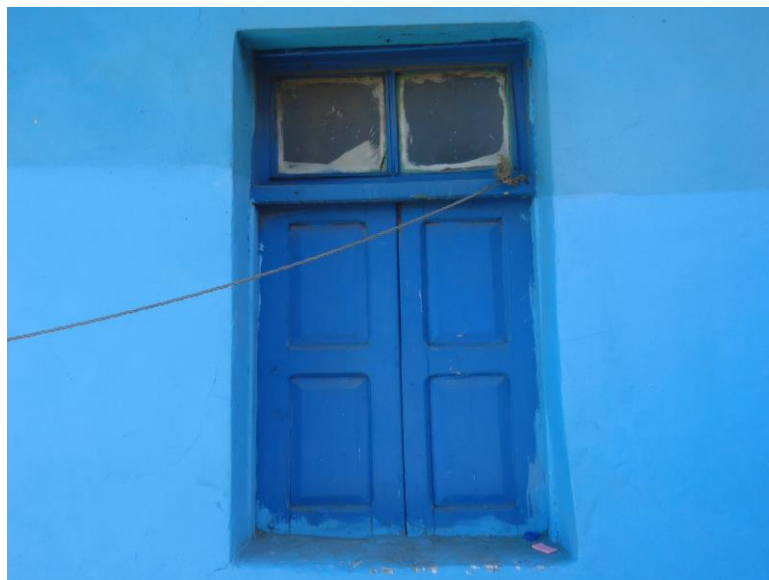
Figure 18: Wooden window opening located on the first-floor terrace
