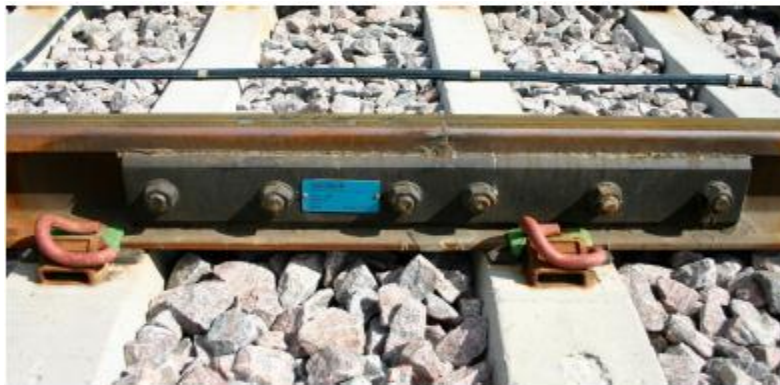
Figure 2.2 Assembled rail joint
