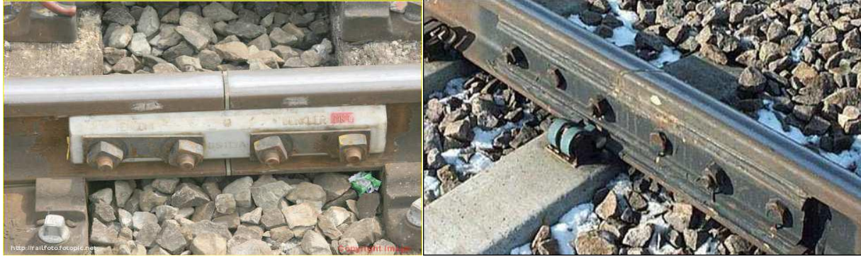
Figure 2.3 Suspended rail joints
