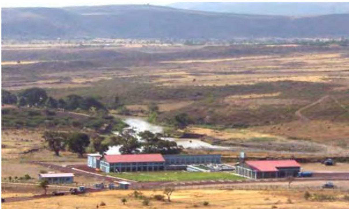
Figure3-11: Adama Water Supply Koka Treatment plant
