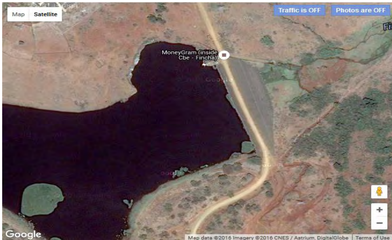
Figure 2.4 Fincha`a rock fill Dam
