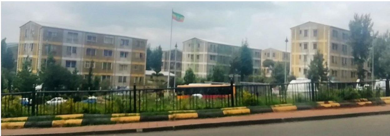
Figure 3-4 Picture of the site showing the Houses in Mickey Leland Site (Researcher 2022)
