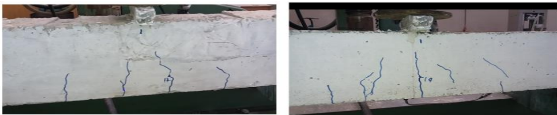
Figure 5-14 state of beams after preloading
