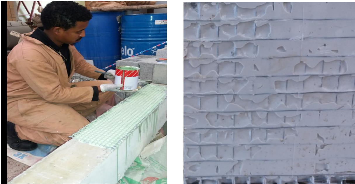
Figure 3-12 Laminating the bonded wiremesh with epoxy
