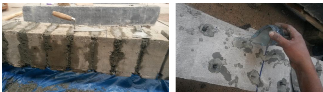
Figure 3.11: Fill the Drilled and Grooved after Placing the Stirrups
