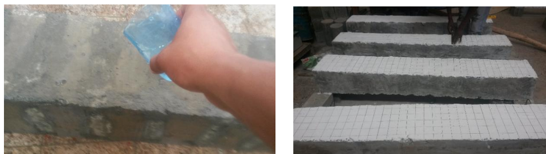
Figure 3.11: Fill the Drilled and Grooved after Placing the Stirrups
