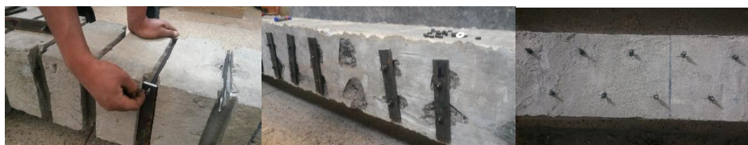
Figure 3.10: Stirrups Placed on the Drilled and Grooved
