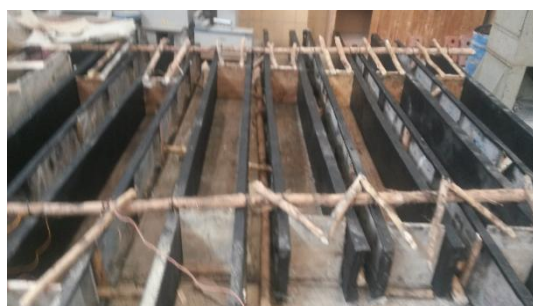
a) Preparation of formwork
