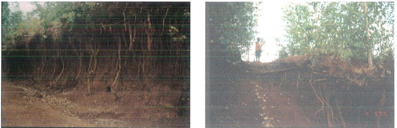
Figure 6.9 Land degradation aggravated by road cut
