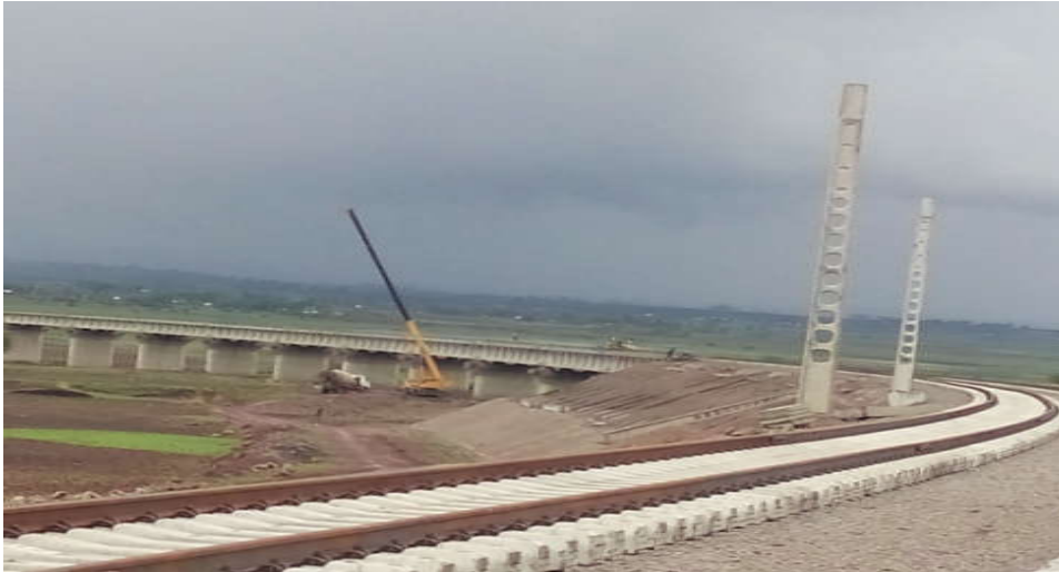
Figure 3-2: Sharp horizontal curve at station 27+600 between Labu and Indode
