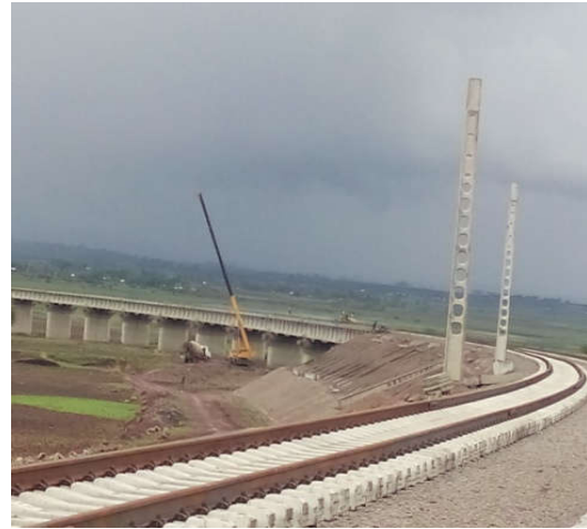
Sharp horizontal curve at station 27+600
