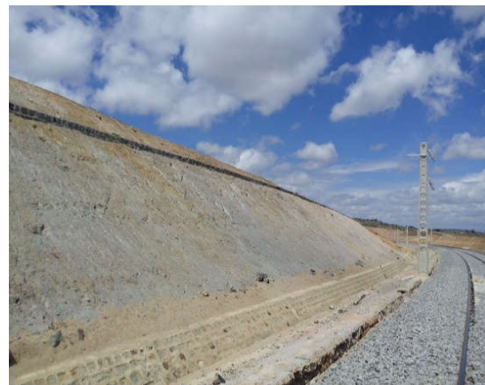
Huge cut at station 95+450
