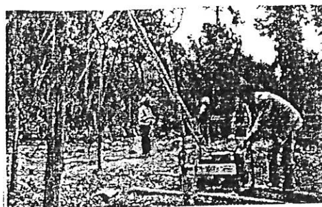
For reliable yield for the aquifer, hand dug well digging continues simultaneously aided by electrical dewatering (pumping water out of the well) pump.
