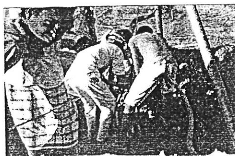
For reliable yield for the aquifer, hand dug well digging continues simultaneously aided by electrical dewatering (pumping water out of the well) pump.
