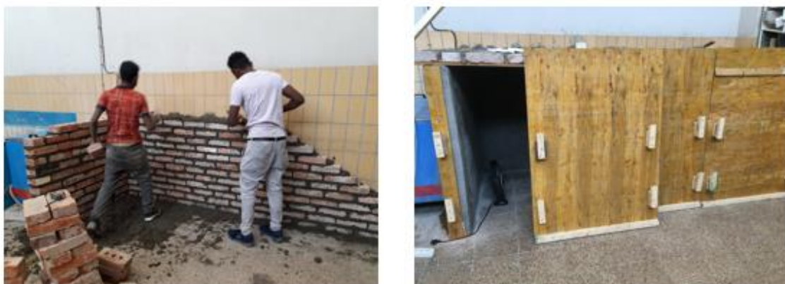
Figure 3.12 Chamber on Progress of Construction
