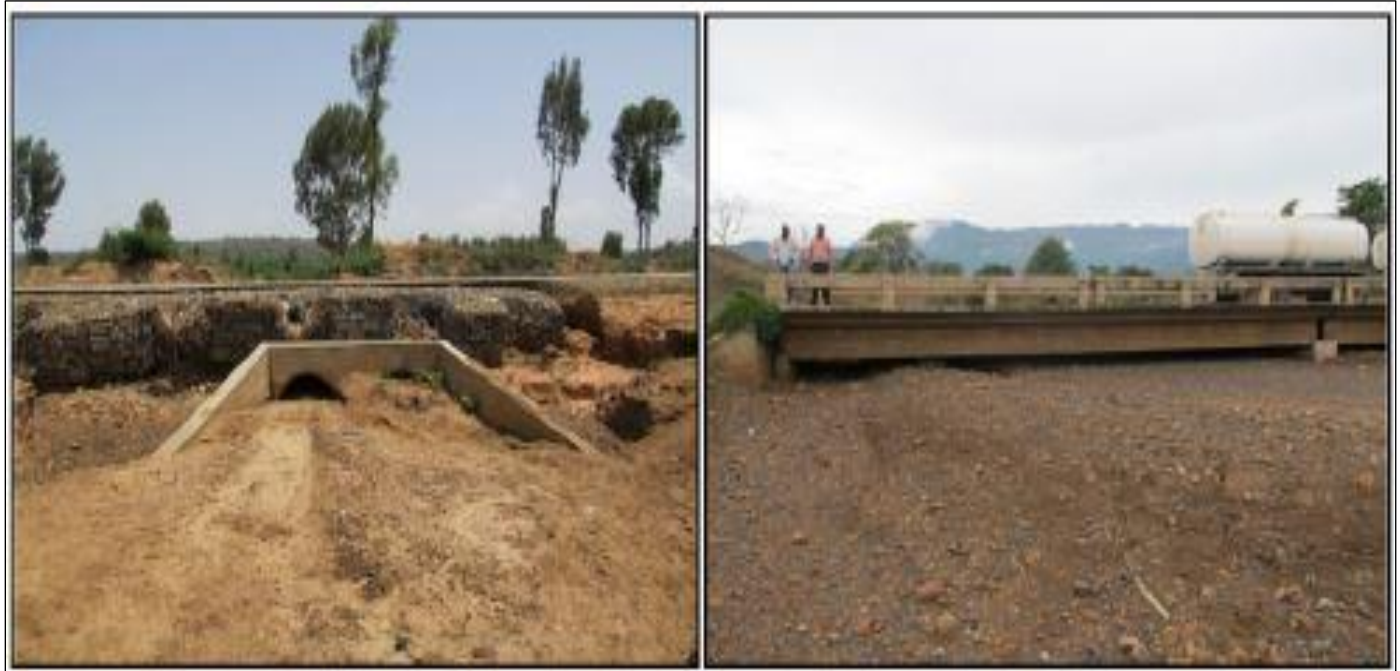
Figure 6 Sedimentation (Source: ERA Drainage Manual 2013)
