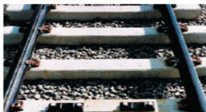
a) Mono-block concrete sleeper
