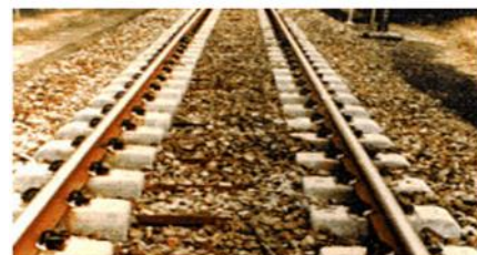
b) twin-block concrete sleeper
