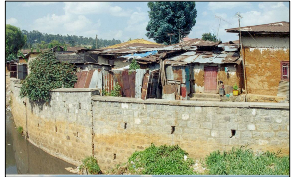
Figure 4.12 flood prevention retaining wall
