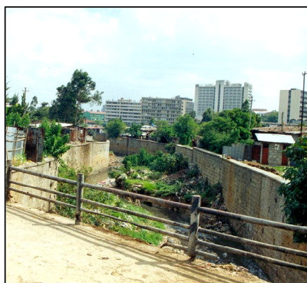
Figure 4.11 flood prevention retaining wall
