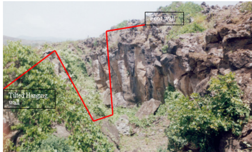
Figure 2.17 View from north to south shows an open normal fault with vertical wall and tilted hanging wall.
