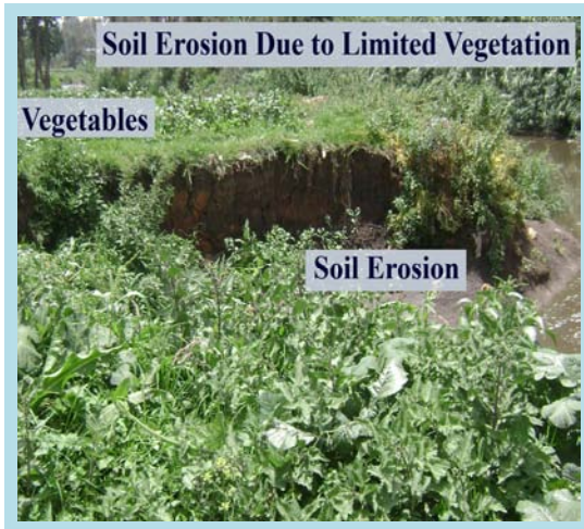
Picture 5.3. Soil Erosion Due to Limited Vegetation Cover
