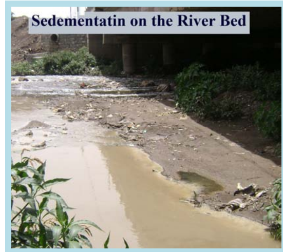
Picture 5.4. Severe Sedimentation of the River in the Study Area
